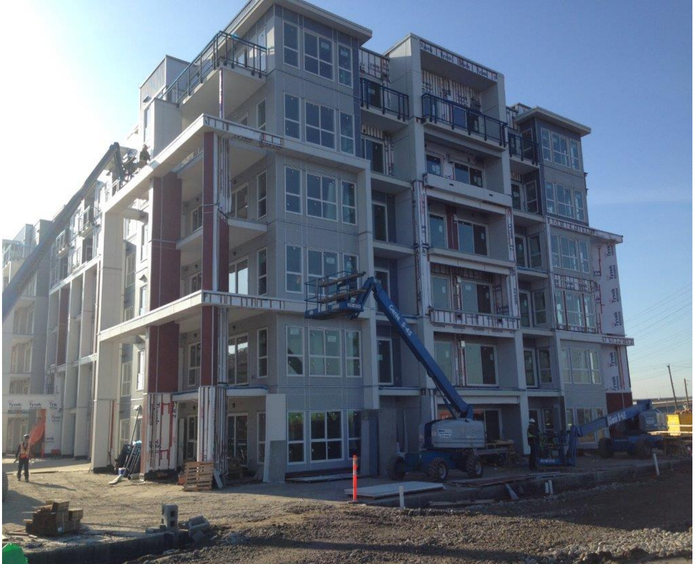
Photo of mid-rise wood frame building under construction.
