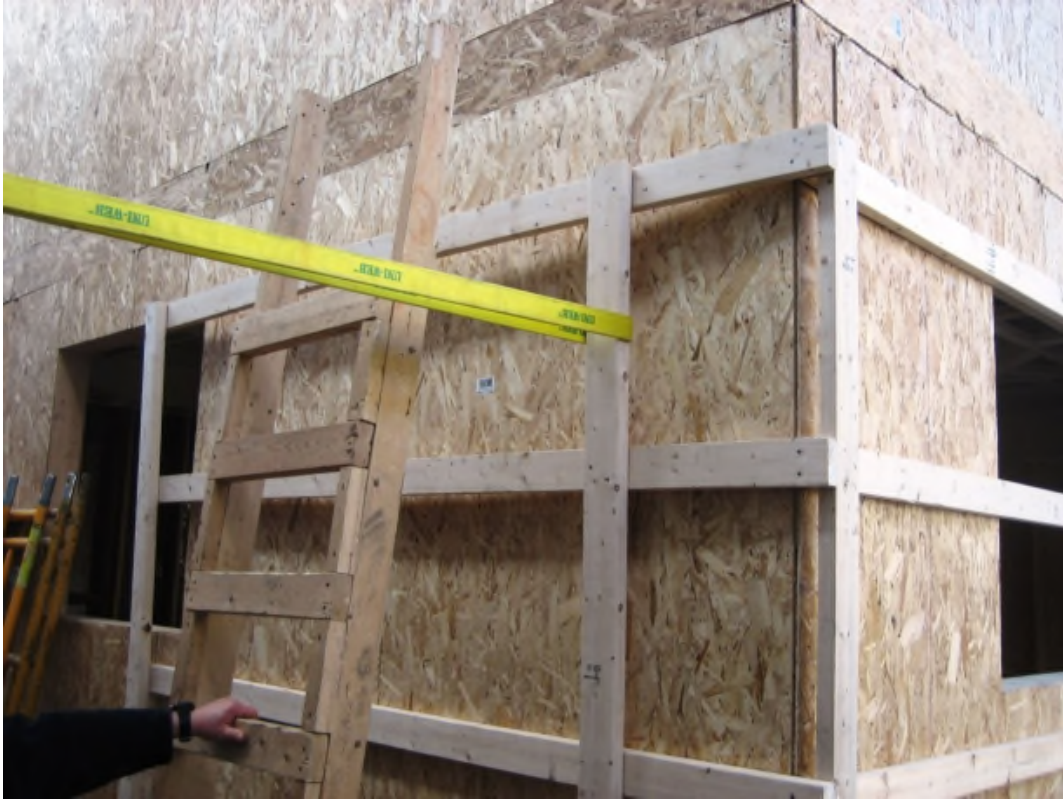
Figure 3: A line was attached to the mid-point of the top- and mid-rail to generate pulling forces on the guardrail.
