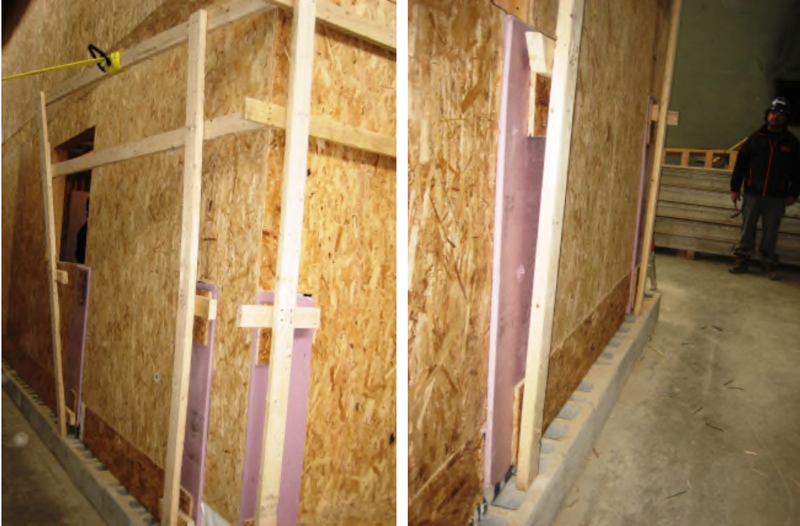
Figure 1: Guardrail setup at Local 183.
