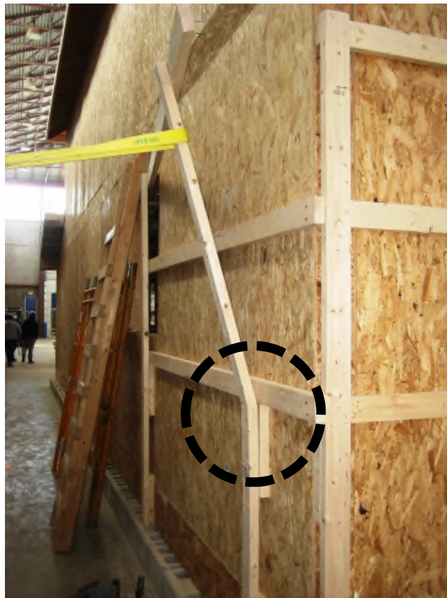
Figure 6: The bottom attachment point failed last.
