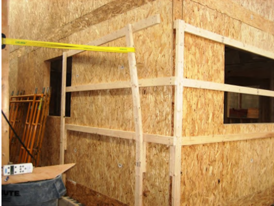
Figure 1: Guardrail setup at Local 183.
