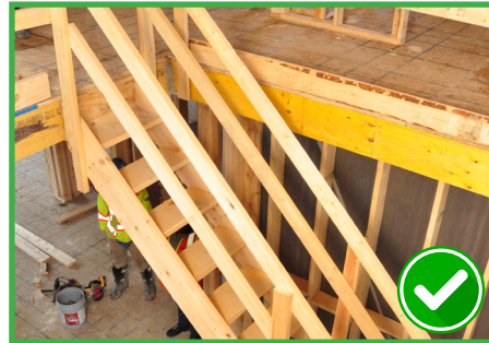
Stairway stringers properly installed
